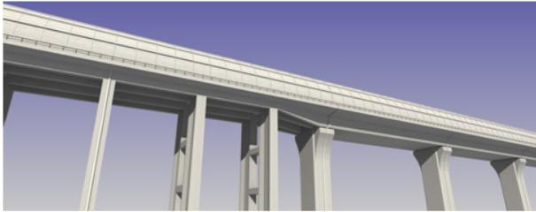
擦り付け部設置案(不連続性を桁部で処理)
